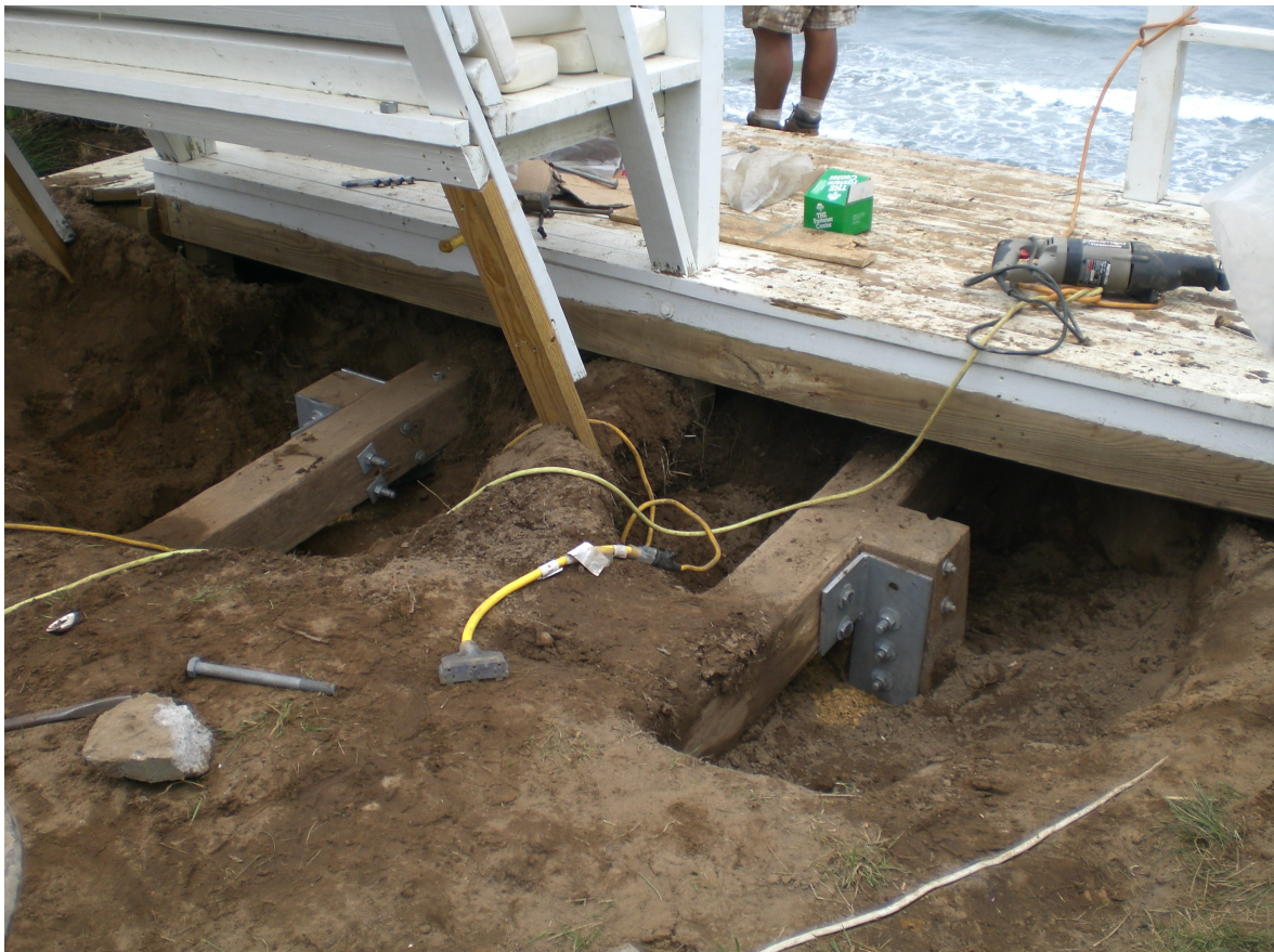
Much of the newly rebuilt and relocated structure was reinforced with steel, including the upper platform grade-beam to post connections.
