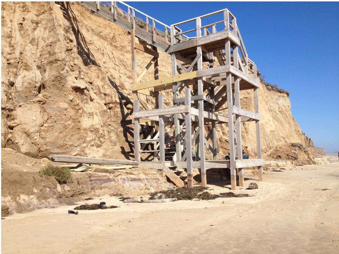
April 2015 – Mud slide from the cliff does not affect the base structure, however it does mean that the upper platform is beginning to cantilever from the cliff edge.
