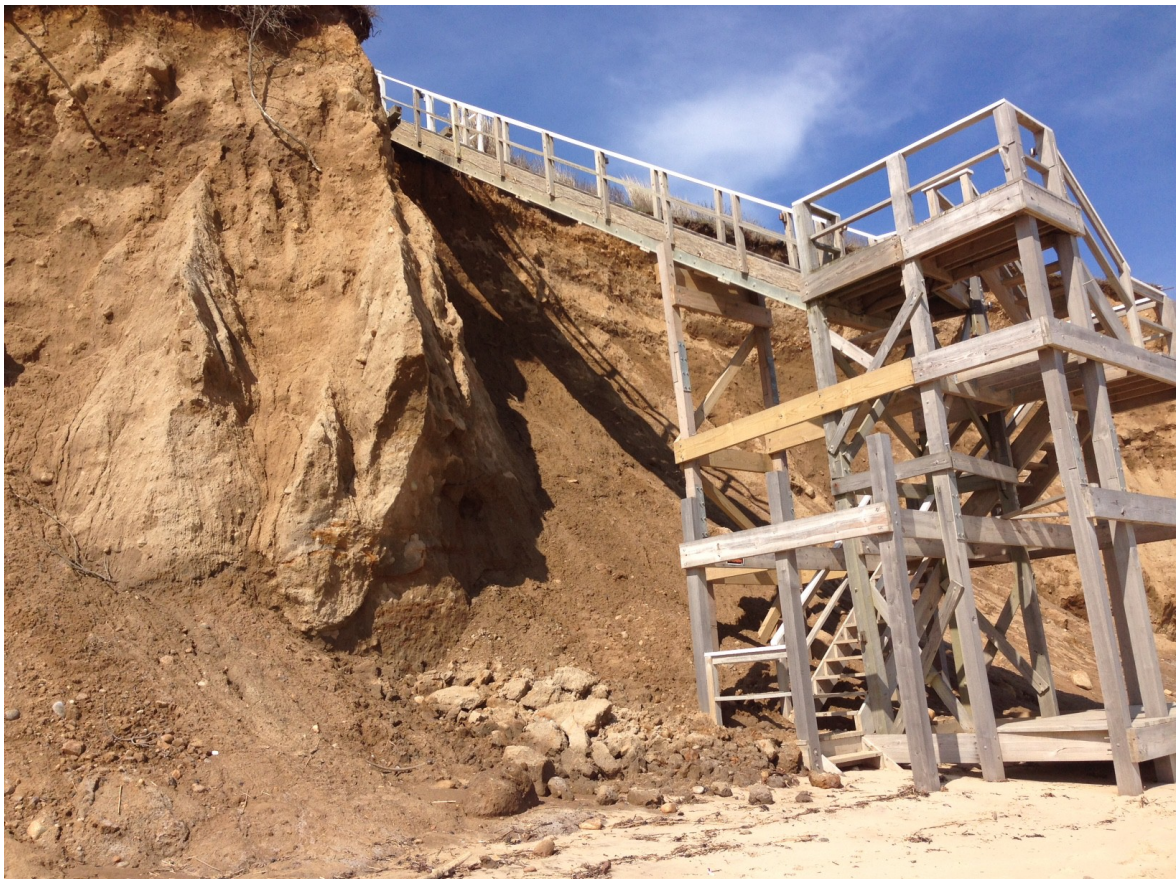
April 2015 – Mud slide from the cliff does not affect the base structure, however it does mean that the upper platform is beginning to cantilever from the cliff edge.
