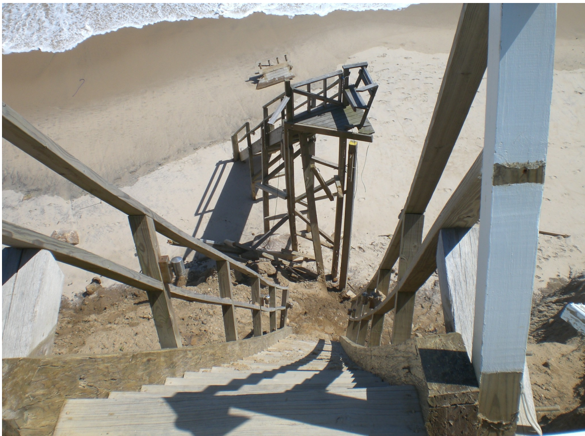
April 2010 - A monsoon rain event and resulting mud slide caused the destruction of the mid-point landing which in turn caused the upper stair to fall and rotate back to the cliff.
