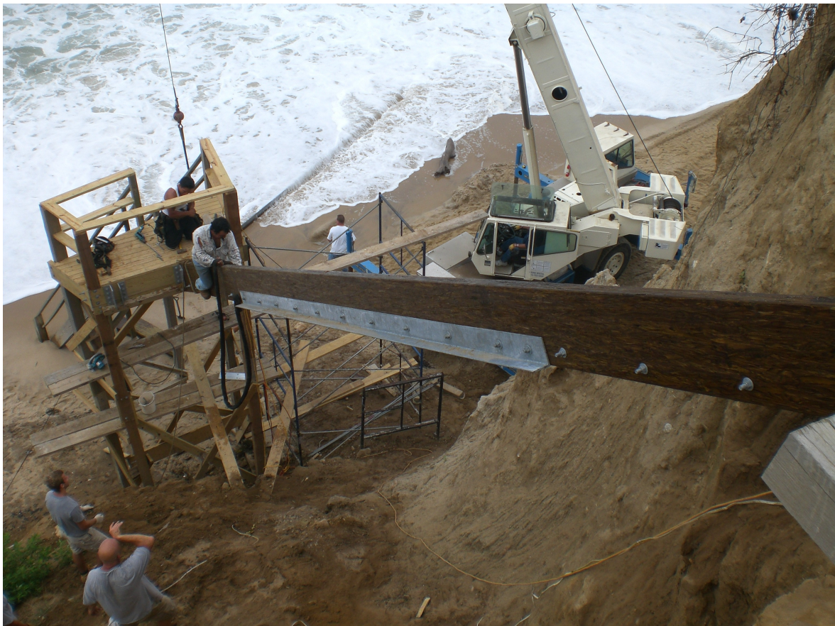
Much of the newly rebuilt and relocated structure was reinforced with steel, including the upper platform grade-beam to post connections.
