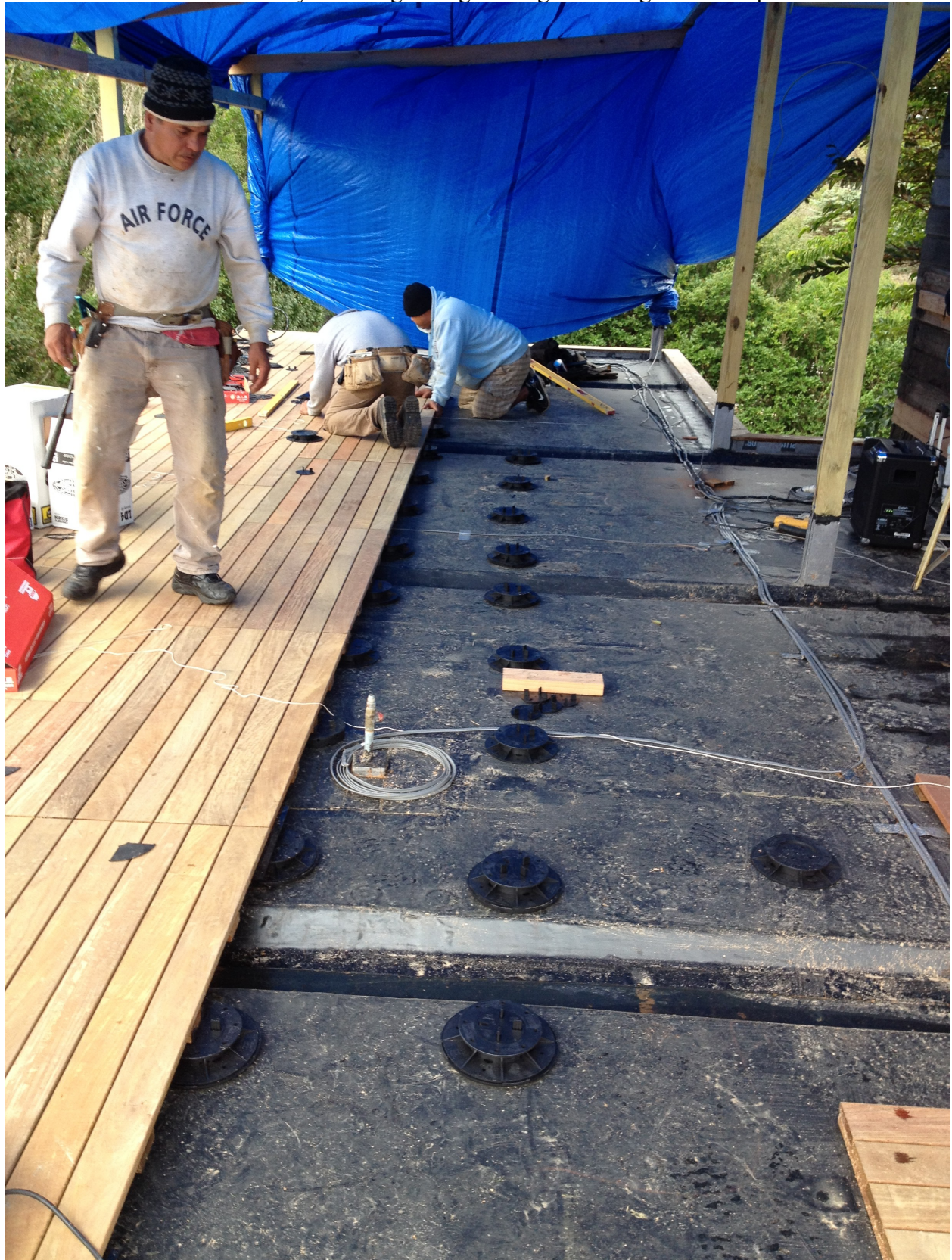
Deck tile installation underway. Drainage troughs designed to align between pedestals.
